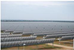
It is a plant with a 150 MW potential per hour, with a surface of 600 hectares. The delegates watched a video that explained which are the main factors for the selection of a place suitable for the construction of such plant: the sun, the presence of water and of transport routes for the transportation of energy. Water is essential because a thermo solar plant is powered by the water cycle.
